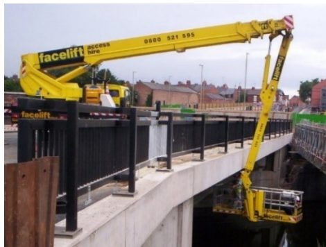
Figure 1-1. Using a cherry picker to inspect a bridge (Facelift Ltd., 2017).
