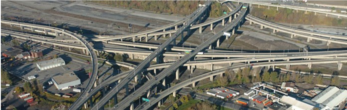
Figure 1-3. Example of highway bridges (Montreal Turcot Interchange) (FOTOimage Montreal, 2017).
