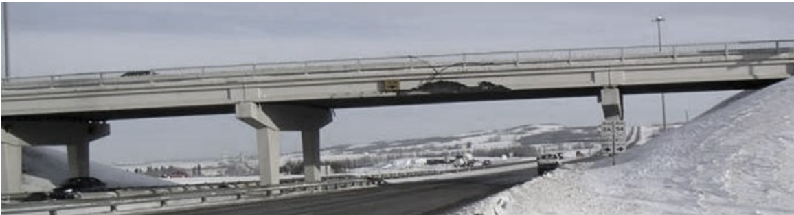
Figure 4-14. Inspected bridge in Alberta, Canada.
