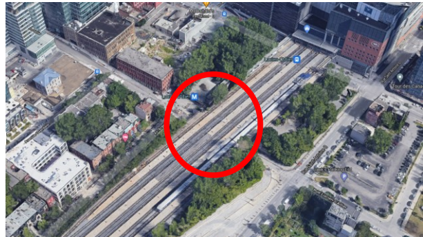
(b) Bridge 2: Lucian L'Allier Street
