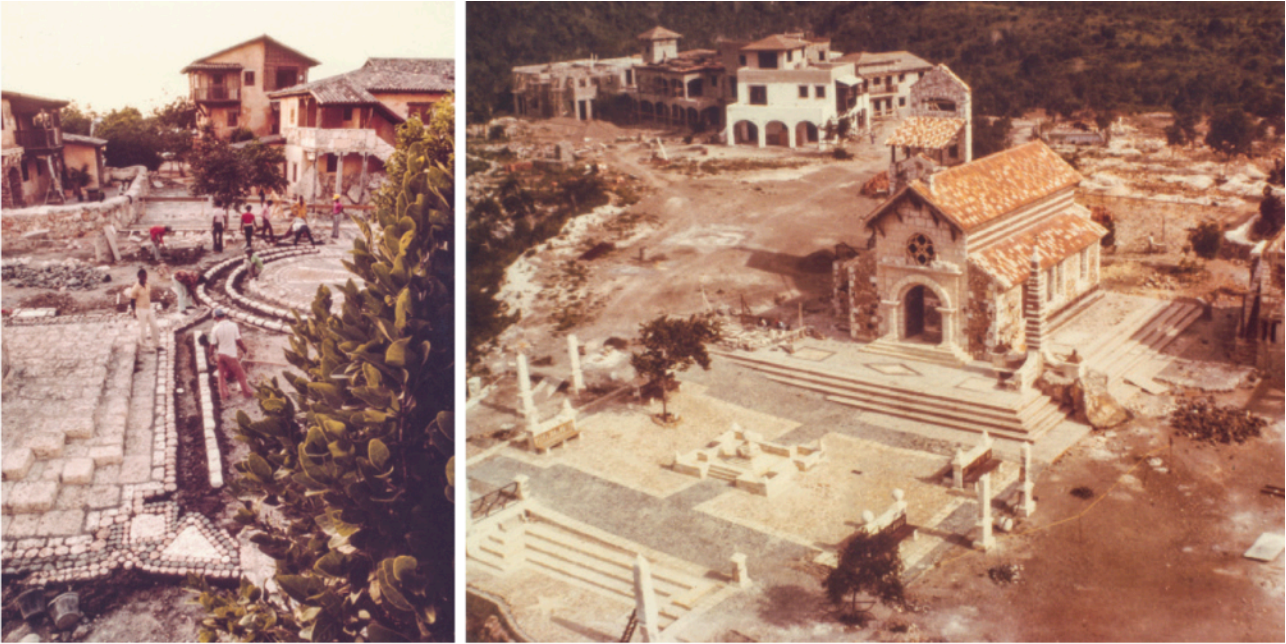
Figure 1: Construction of the first phase of Altos de Chavón, showing the chapel in the foreground; Workers painstakingly lay out the cobble streets, photographed in the late 1970s. Image courtesy of Casa Life Magazine, 2017.
