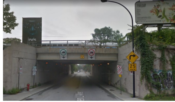
(b) Bridge 2: Lucian L'Allier Street
