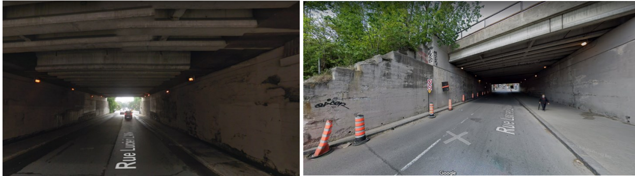
Figure 6-19. Images of the bridge
