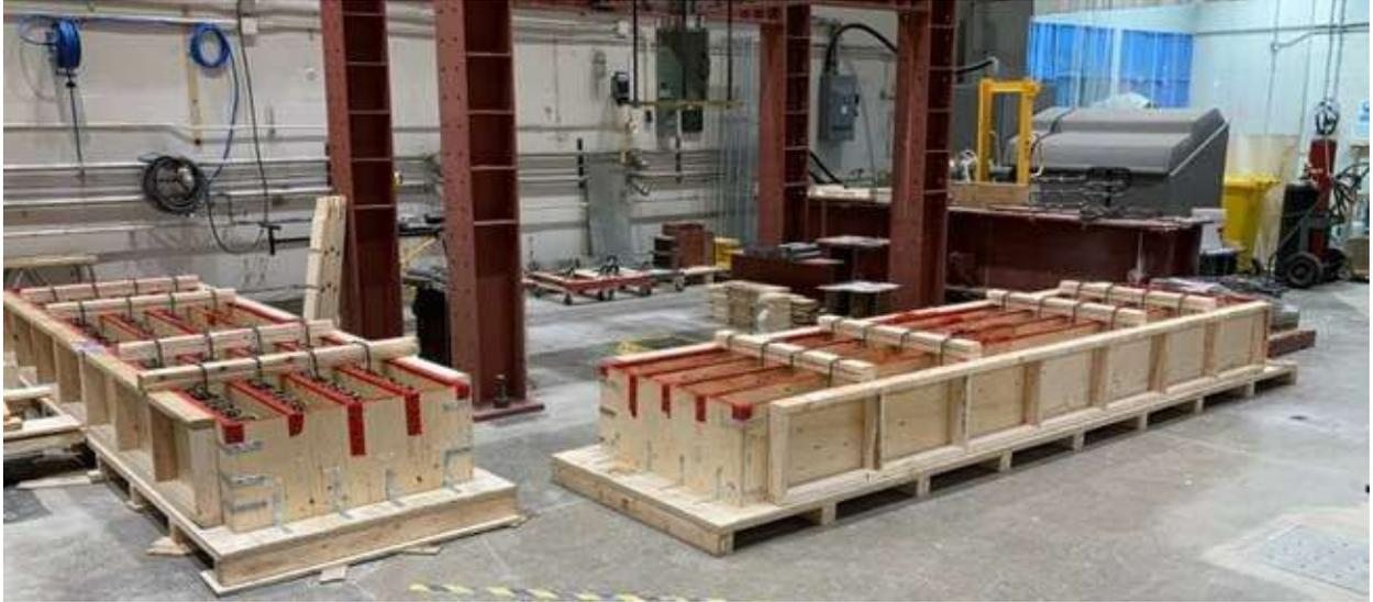
**Figure A.5** Preparing and levelling the formwork for the concrete pouring
