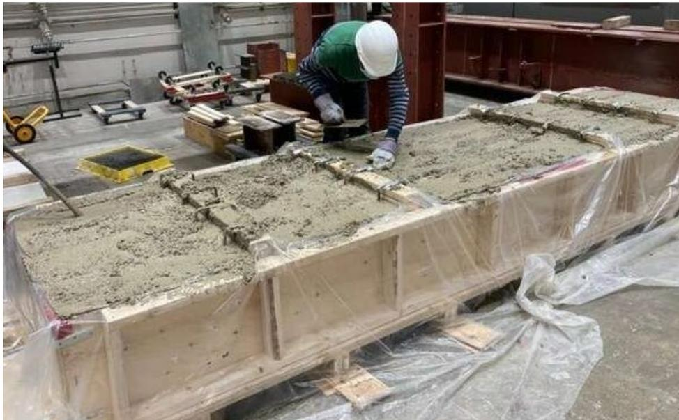
**Figure A.8** Careful finishing of the top concrete surface using trowels
