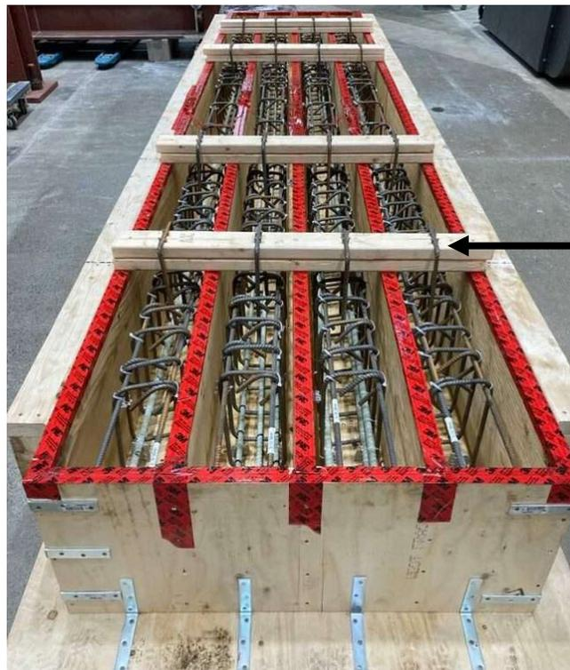
**Figure A.4** Preparing the formwork for the concrete pouring by fixing the top steel hooks
