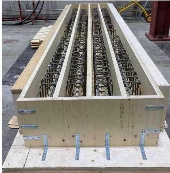
**Figure A.3** Placing the cages inside the formwork
