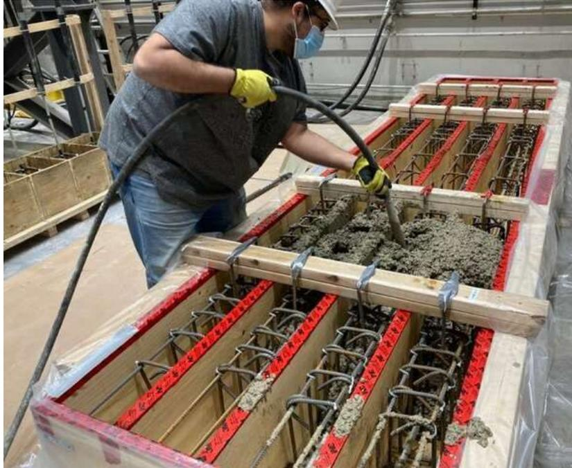
**Figure A.7** Vibration of poured concrete using the electric vibrator
