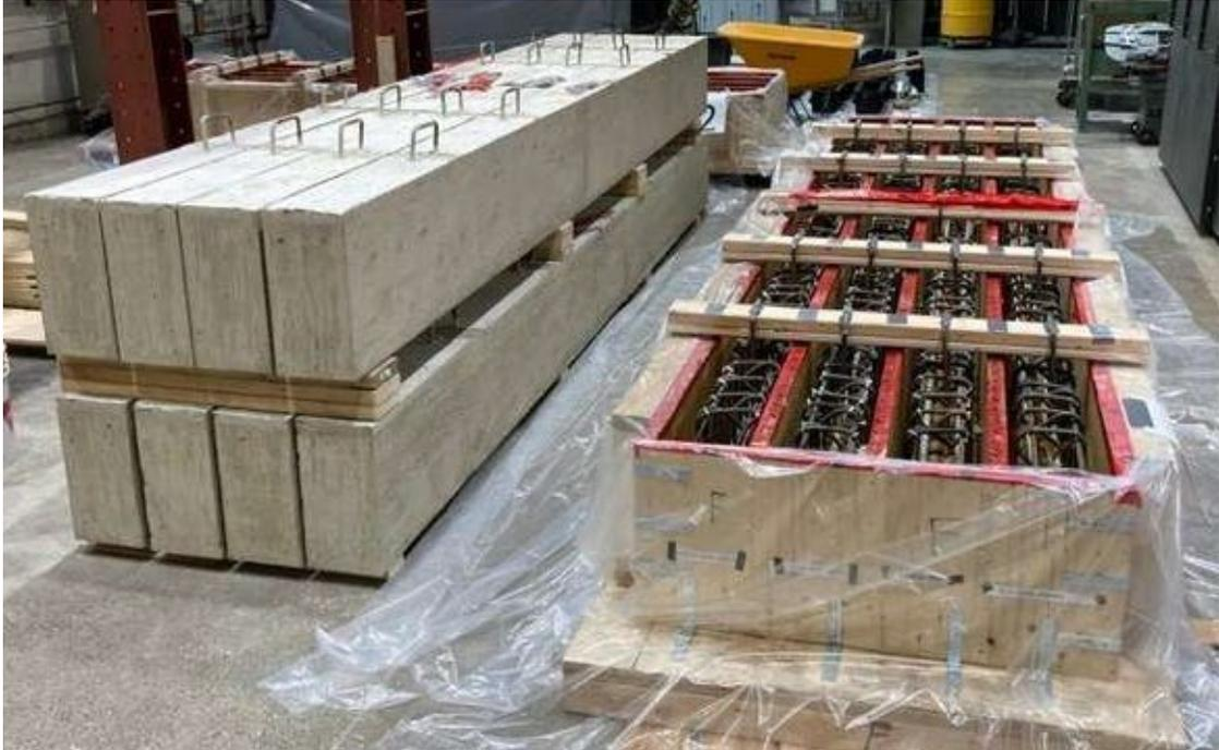
**Figure A.13** Stacking of the concrete beams after disassembling of the formwork
