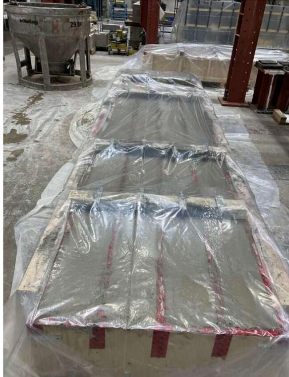
**Figure A.11** Covering the concrete surface with a plastic cover for curing
