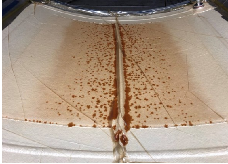
Figure 66. Membrane leakage in the 3 rd trial
