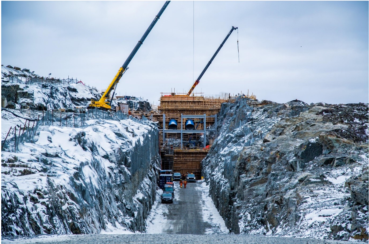
10. Currently dry, this is where the Innuksuac river will eventually flow once the project is in operation. The 7.5-megawatt project is expected to reduce greenhouse gas emissions by 700,000 tonnes over 40 years. It's the first initiative of its kind in Quebec, created in collaboration between Inuit-led Pituvik, Innergex (a Quebec renewable energy company) and Hydro Quebec.
