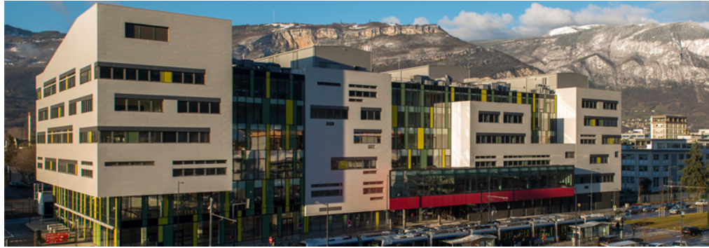
Figure 2.1: GreEn-ER: a building for energy learning and research.
