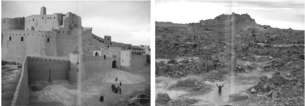
Figure 4: Arg-e Bam before the 26 December 2003 earthquake (left) and after the earthquake (right). (Left photo by M. Eslami Rad, Ministry of Housing and Urbanization. Right photo by A. Shahroodi, Nashravaran Journalistic Institute)
