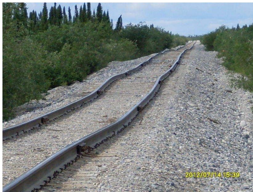
Figure 2.5. Vertical deformation of railway track constructed on a highly compressible peat (De Guzman and Alfaro 2017).
