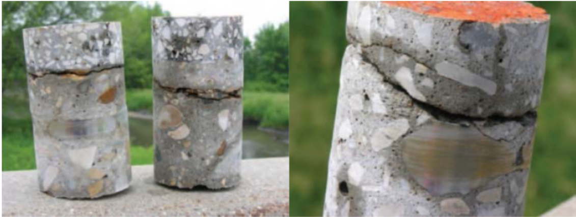
Figure 2.7 Delamination observed in cores (Gucunski & National Research Council, 2013)
