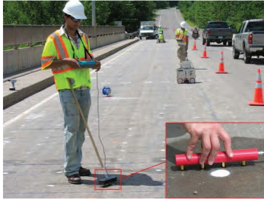
Figure 2.19 Electrical Resistivity testing using a Wenner probe (Gucunski & National Research Council, 2013)
