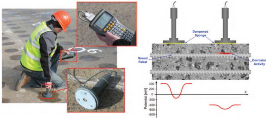
Figure 2.18 (a) GPM Testing and (b) GPM Principle (Gucunski & National Research Council, 2013)
