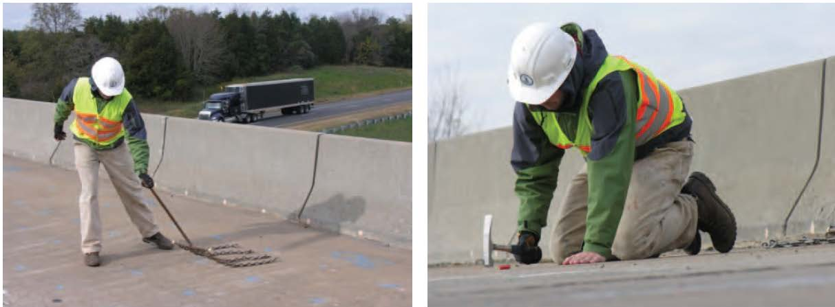
Figure 2.22 Chain Dragging (left) and Hammer Sounding (right) (Gucunski & National Research Council, 2013)
