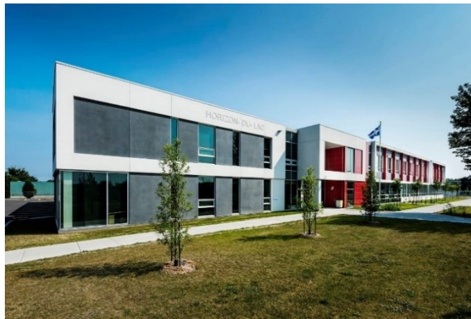
Figure 6-9: Horizon-du-Lac school building
