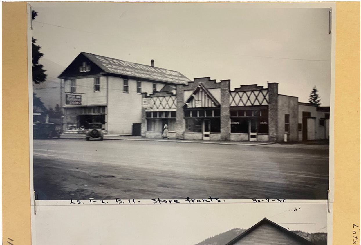
Figure 13. Store Fronts of Block 11, Lots 1-2, September 30, 1937, V488/I.A./PA/Block11, Lot1-2, Parks Canada fonds, Whyte Museum, Banff, AB.
