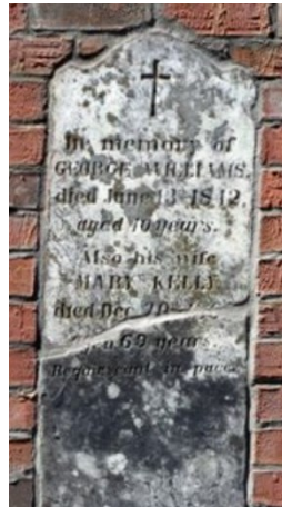
#155-George Williams monument mounted on the wall and before cleaning.
