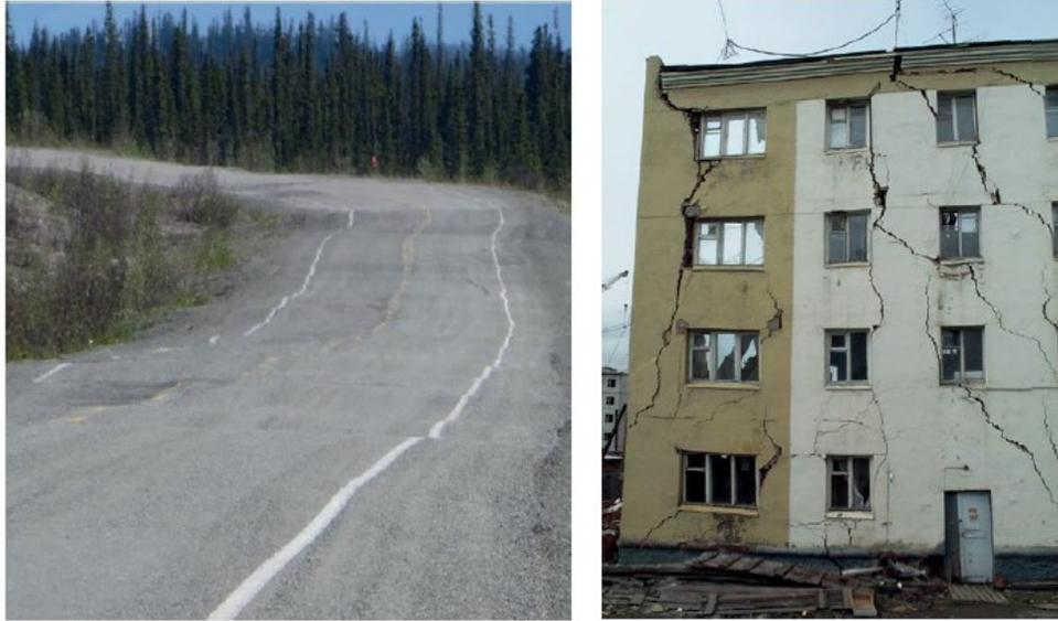
Figure 1-1 Construction issue in permafrost regions due to degradation (Hjort et al., 2022).
