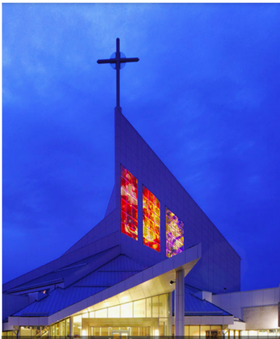
Figure 3a. Sarah Hall, Lux Gloria , 2011. Airbrushed glass panels with embedded solar cells and laminated dichroic glass, 1128 x 365 cm each. View Source
