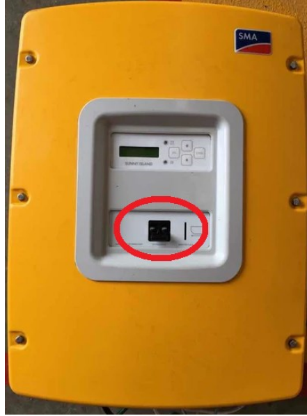
Figure 4-18: Disconnect Switch on the casing of SI
