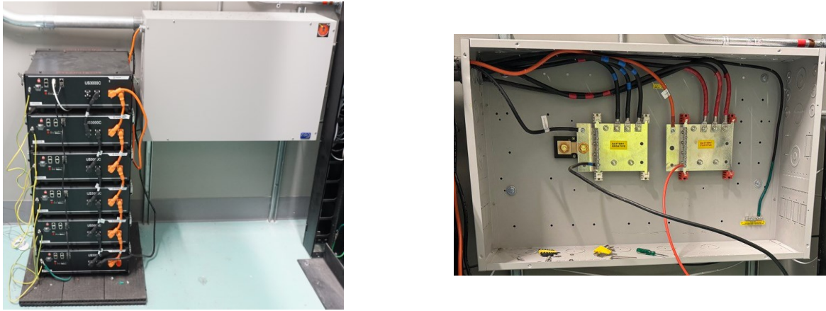
Figure 4-4: Stationary Battery and DC Splitter Box
