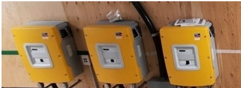
Figure 3-4: Battery inverters (Sunny Island 1, 2, and 3)
