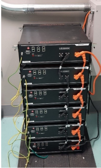
Figure 3-3: 6 units of Pylontech - US3000C connected in parallel
