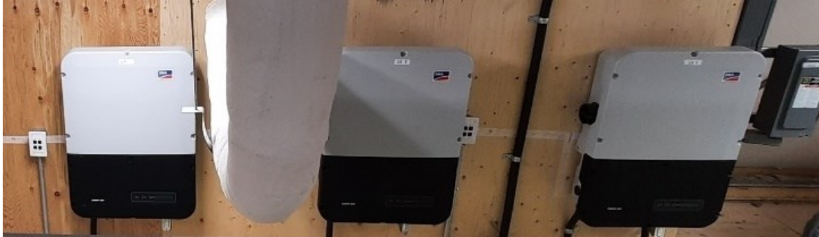
Figure 3-2: PV inverters (Sunny Boy 1, 2, and 3) at FBL.
