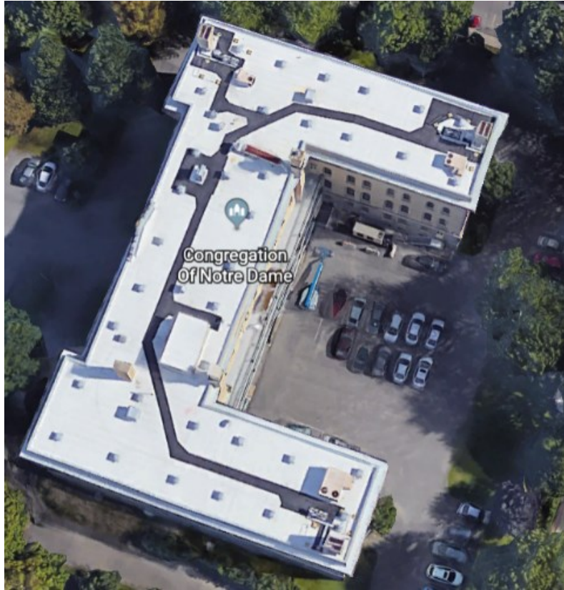
Figure 1.2: A U-shaped building in Montreal.
