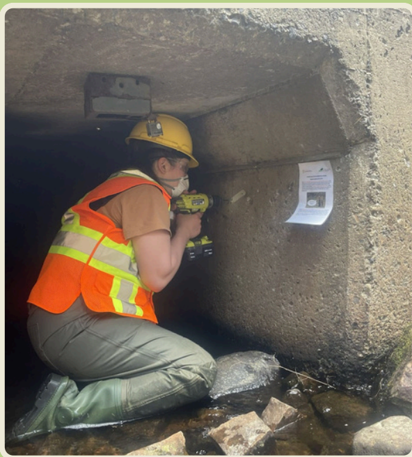
Figure 6. Researcher installing a camera in a culvert (Photo credit: Daphné Mary, 2025)
