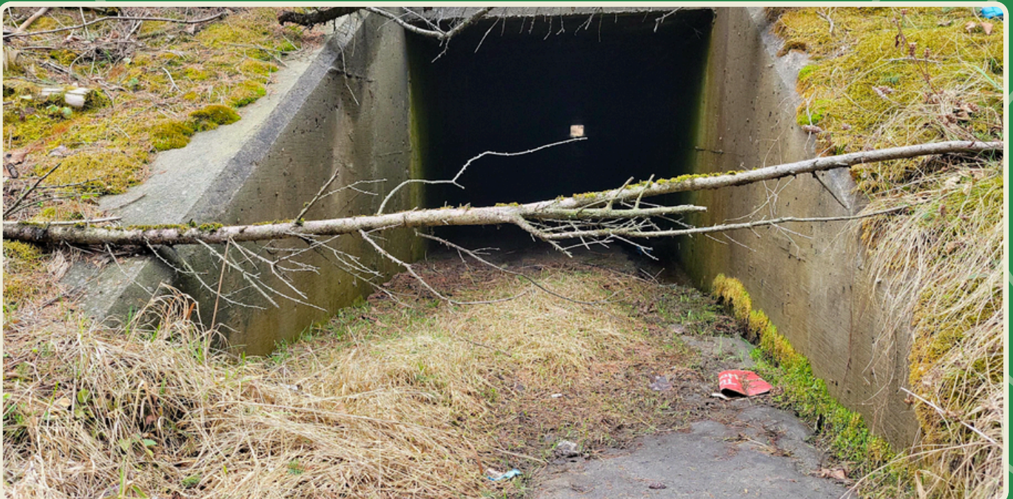
Figure 3. Example of a structure designed for water passage under the roadway that can be used by animals to cross under the road. (Photo credit: Amanda-Faith G  linas-Noble, 2025)
