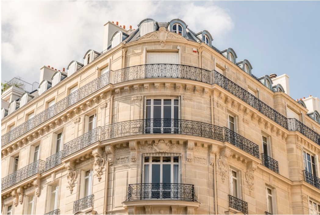
Figure 20. Pierre Emmanuel Faivre, Iconic wrought iron balconies on a Haussmann apartment building. Photo: Stock Photos from Pierre Emmanuel Faivre/Shutterstock.
