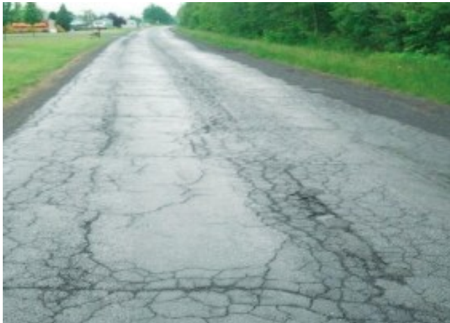
Figure 15: Cracking Example [104]
