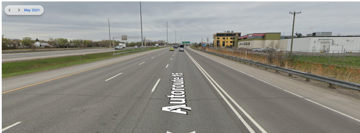
Figure 33: Autoroute 15 - May 2021 (Source: Google Earth®)
