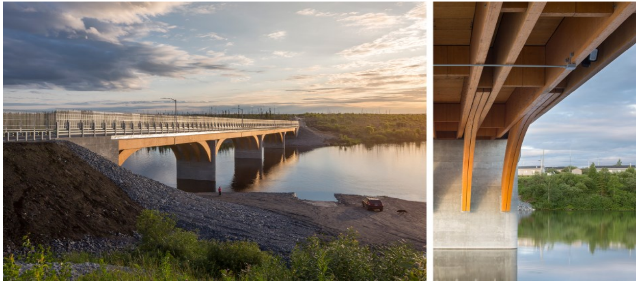
Figure 2.9 Mistissini Bridge in Quebec [28]
