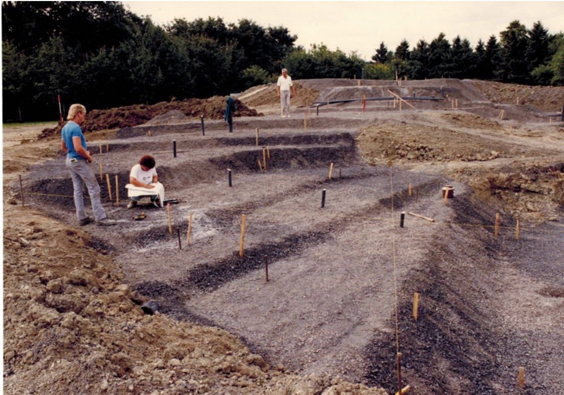
Figure 11. Ground preparation for the installation of waterfall and garden, Jardin botanique de Montréal, 20.08.1987. (Photo credit: Archives – Jardin botanique de Montréal)
