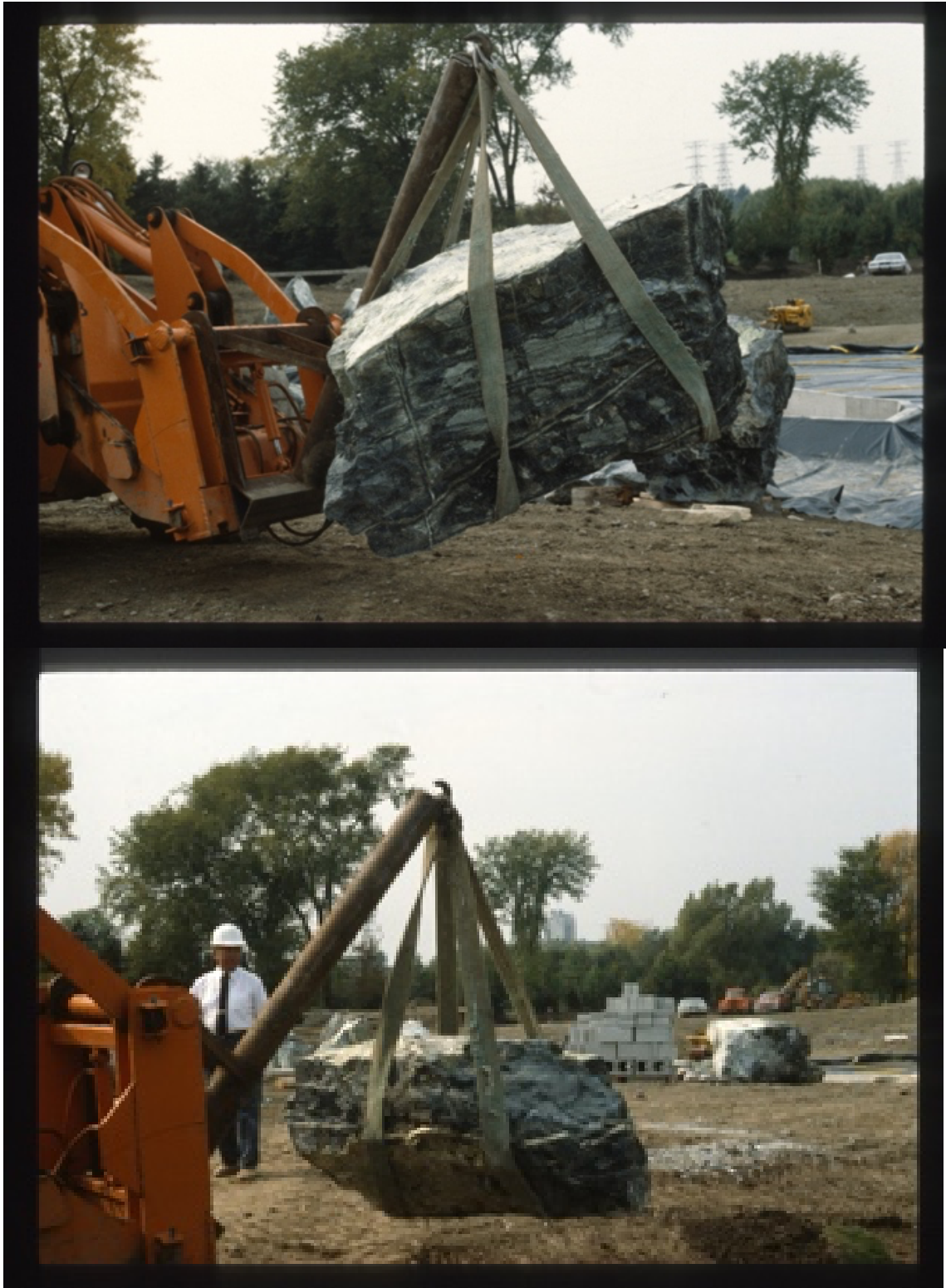
Figures 19 and 20. Moving stones into the garden via crane. In figure 20 Ken Nakajima is overseeing the positioning, Jardin botanique de Montréal, 25.09.87. (Photo credit: Archives – Jardin botanique de Montréal)
