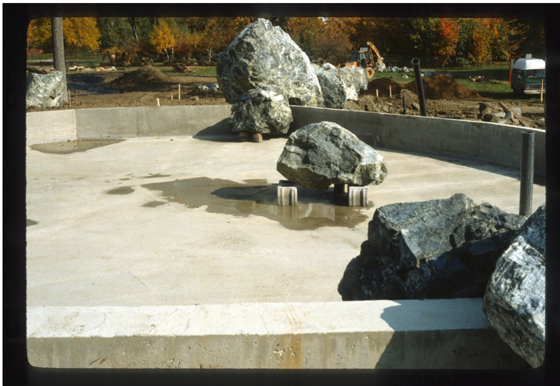
Figure 25. Support structures for large stones placed in the pond at the top of the waterfall, 06.10.1987. (Photo credit: Archives – Jardin botanique de Montréal)
