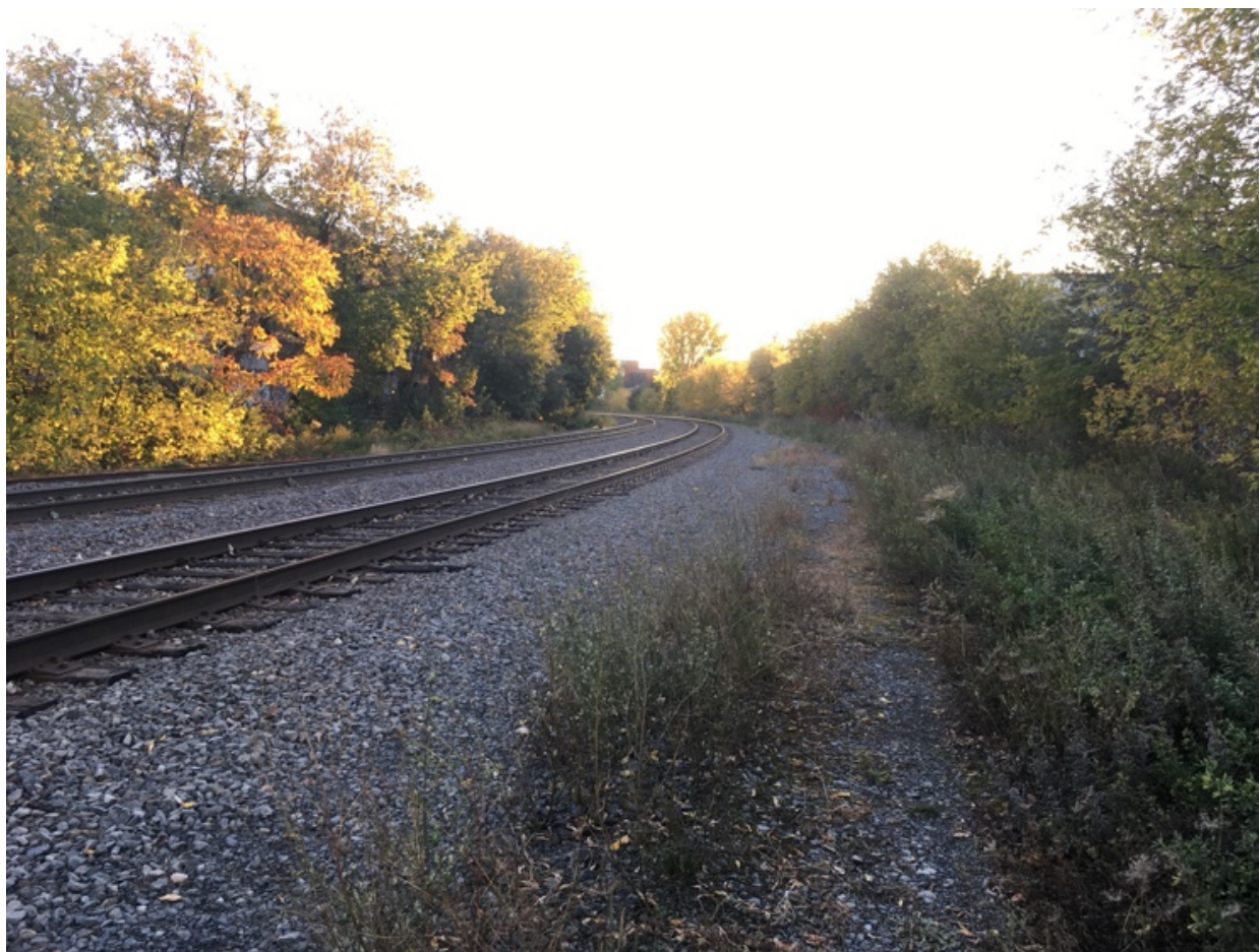
Figure 75. Train tracks and path running along the southern border of the Home Depot parking lot, 11.10.2020.
