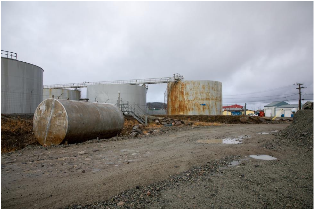
Caption: Rusting diesel tanks in Inukjuak mark the end of an era. Before the community transitioned to clean hydropower, these storage tanks held millions of litres of diesel fuel needed to heat homes and generate electricity.
