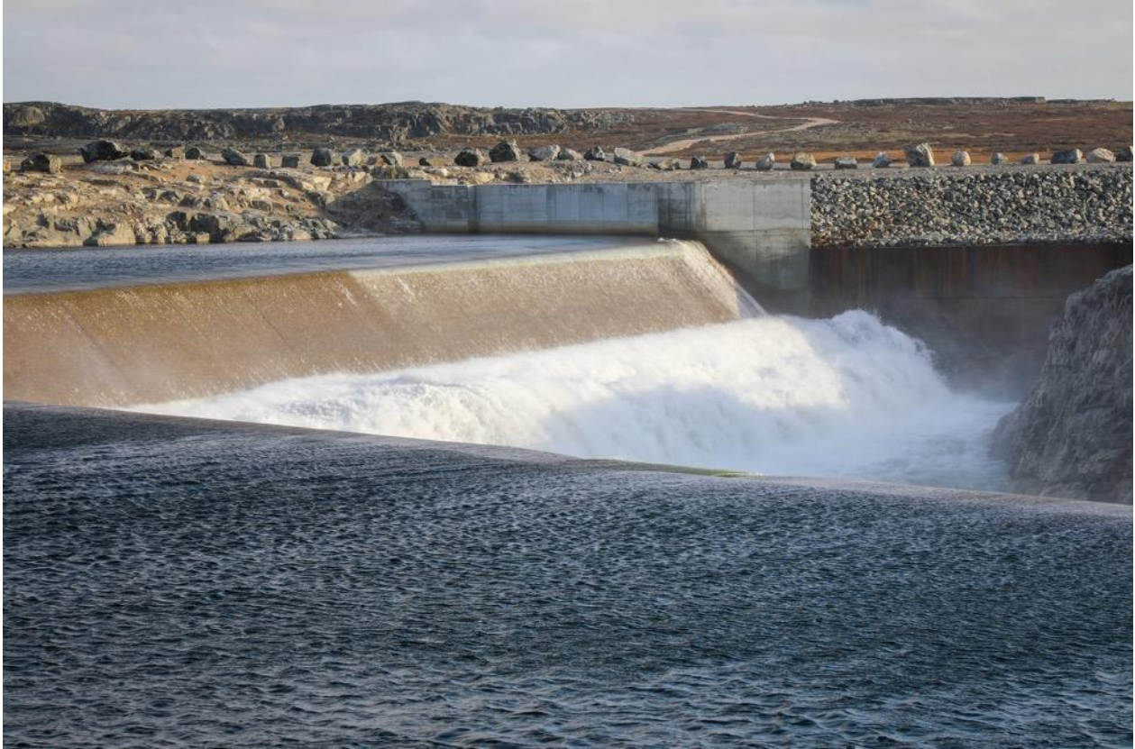
Caption: The Innavik Hydro facility on the Innuksuak River, October 2024. This 7.5-megawatt, Inuit-owned facility is the largest off-grid hydropower project in Canada. Photo by Lina Forero as part of a documentary on Inukjuak's clean energy transition, created for her master's thesis with Concordia journalism professor Aphrodite Salas.
