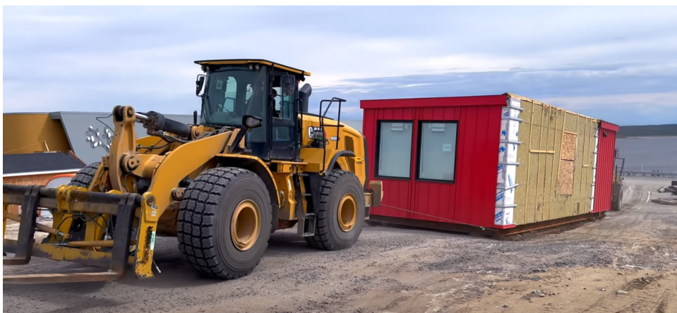
Figure 19: On-site placement of prefabricated housing module using heavy machinery
