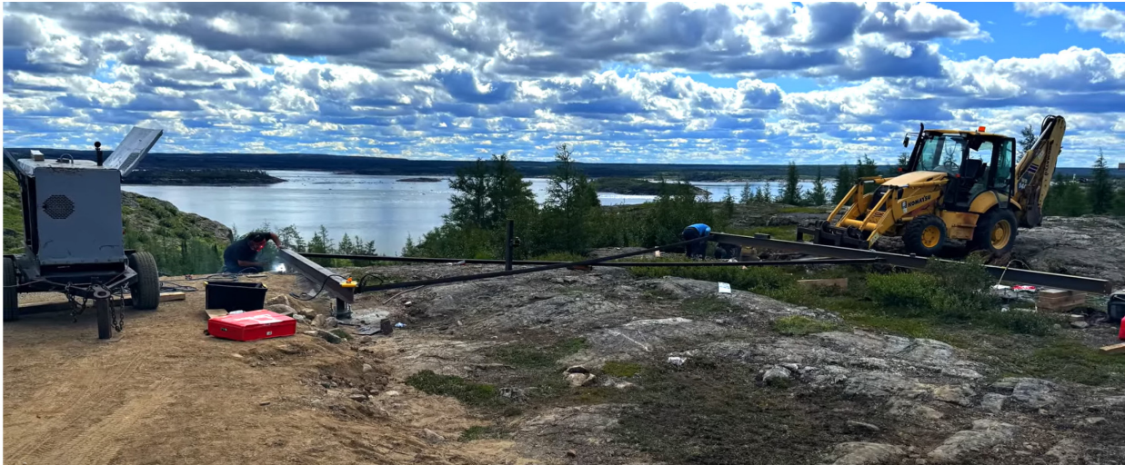
Figure 25. A5 installation of one prefabricated unit
