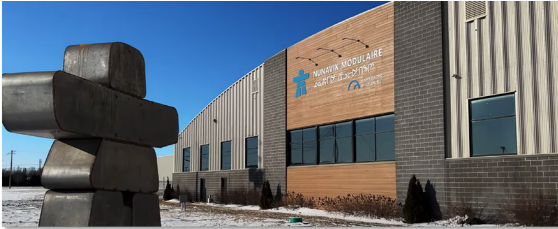
Figure 11: Nunavik Modular factory facility in Napierville, Québec.
