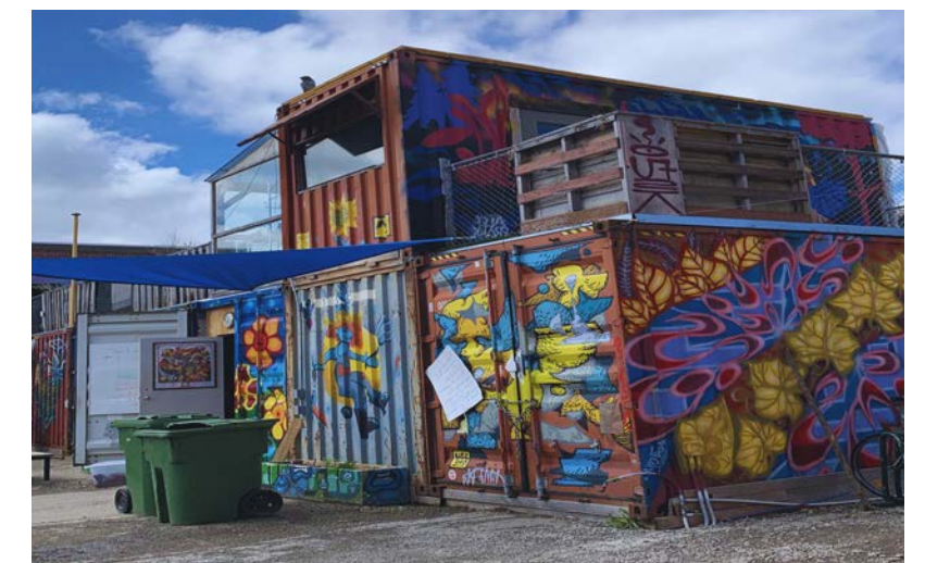
Bâtiment 7, outdoor kitchen part of the Greenhouse (lot 5).
