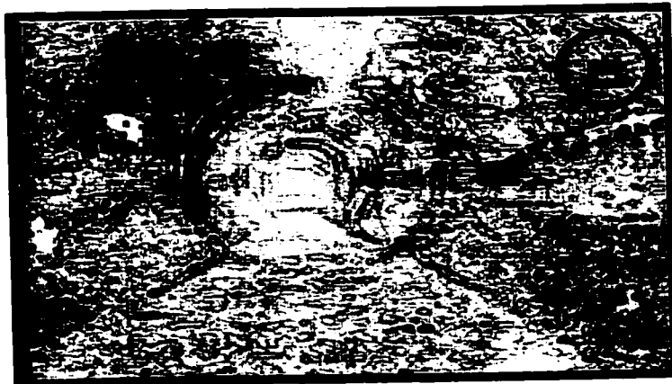
Figure 3-14: Edge Detected Image of Cracks
