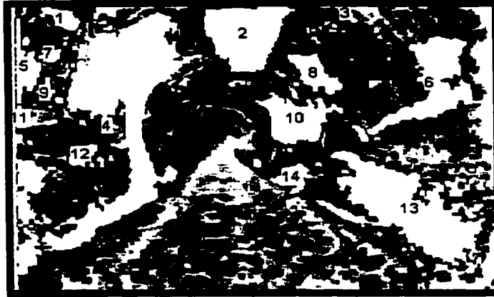
Figure 3-60: Segmented Image of Cracks
