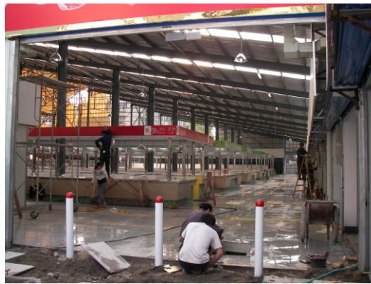
Figure 5.10 Floor is replaced. (Yingbin Caishi, 2007)
