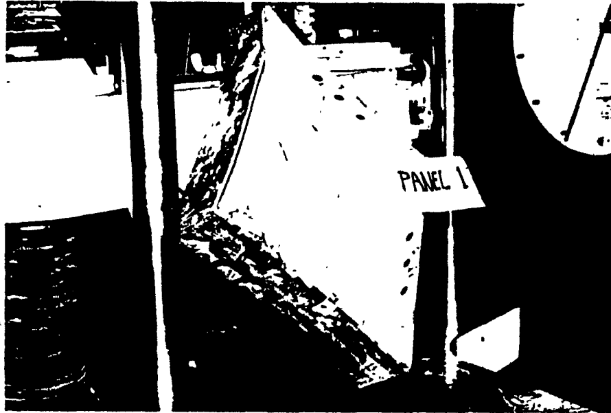
FIG. 4.6 PANEL NUMBER 1 AT COLLAPSE
