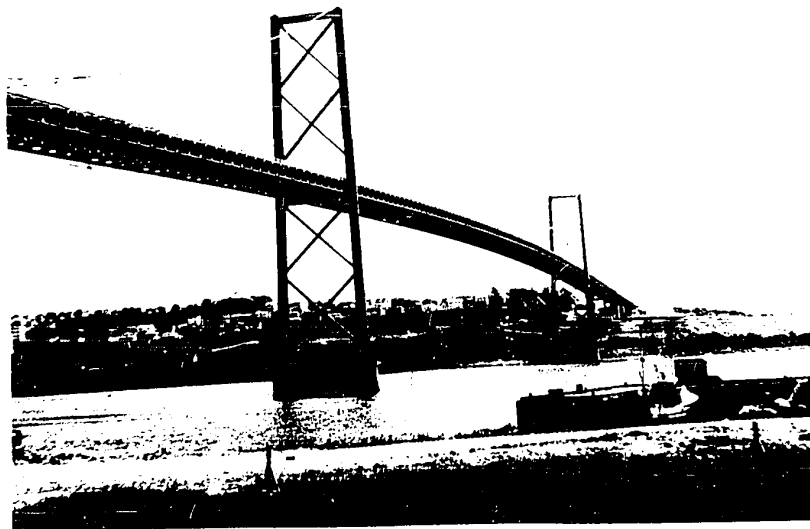
FIG. 11.20 THE COMPLETE VIEW OF THE A. MURRAY MACKAY BRIDGE
