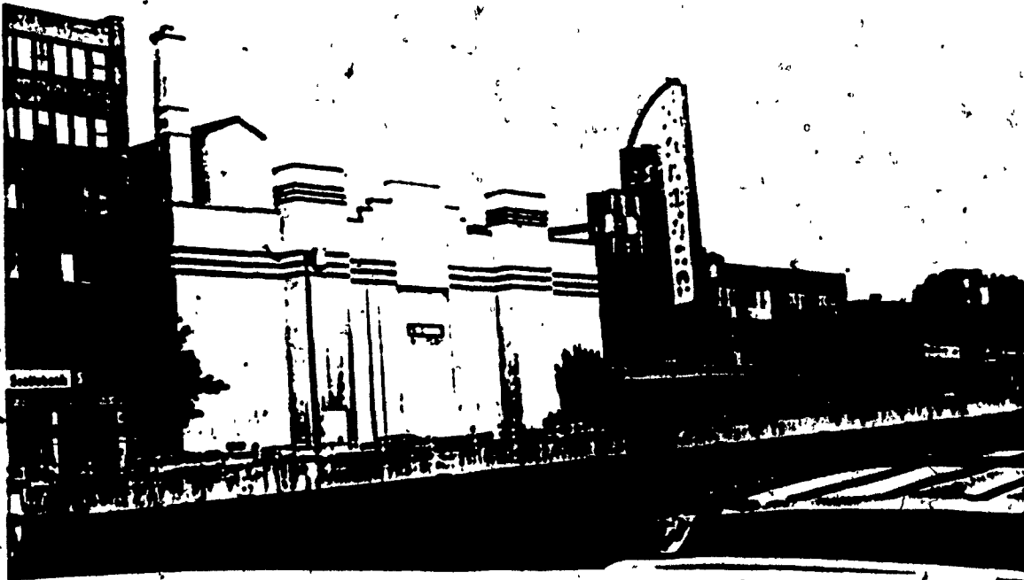
Fig. 61 SNOWDON: Main facade; Photograph by H. Kolomeir. Sept. 1984.
