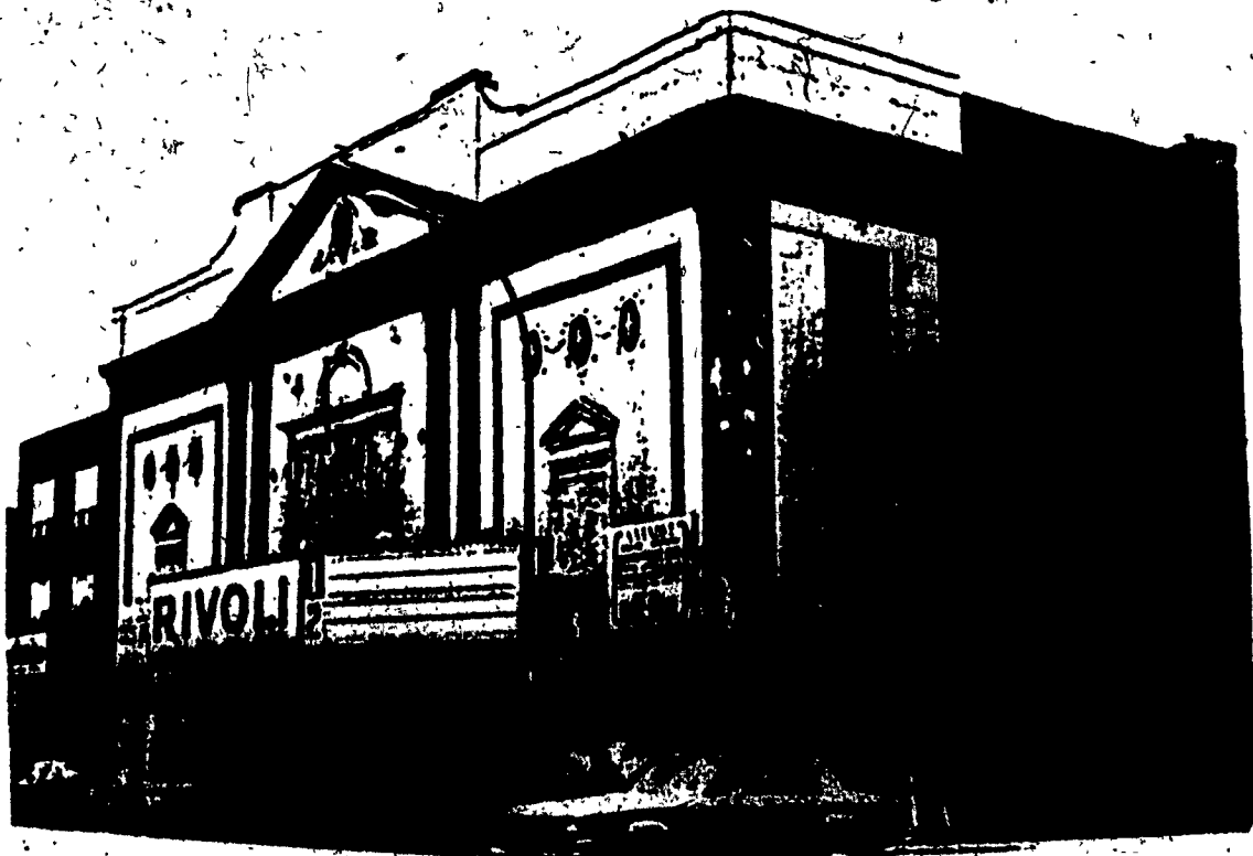
Fig. 7 RIVOLI: Main facade; Photograph by H. Kolomeir. Sept. 1984.
