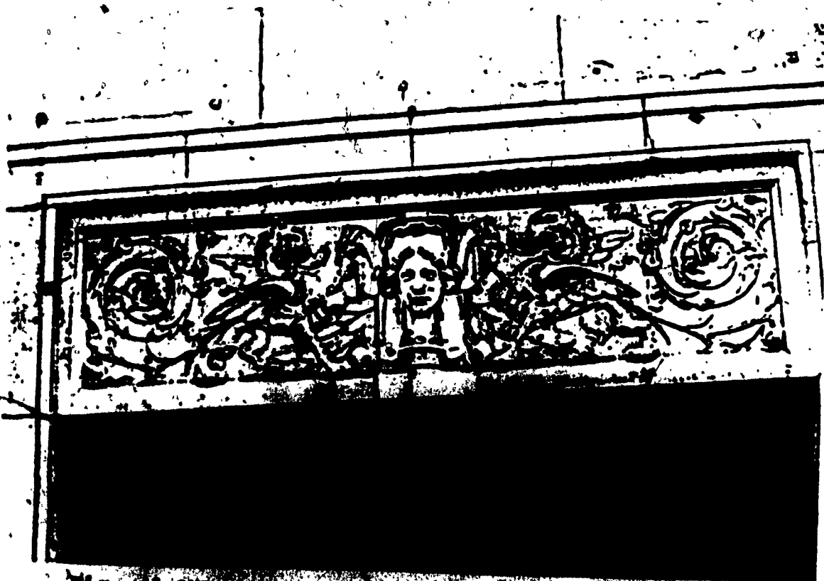
Fig. 41 OUTREMONT: Cast stone panel located over the service doorway; Photograph by H. Kolomeir. Oct. 1985.
