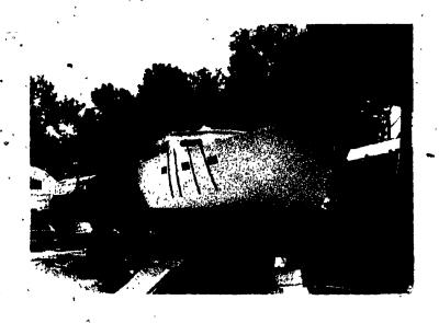
FIG. 1.1 FERRO CEMENT CRUISING YACHTS UNDER CONSTRUCTION
