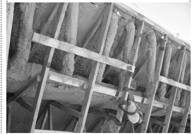
BIPV/T Roof Insulation
