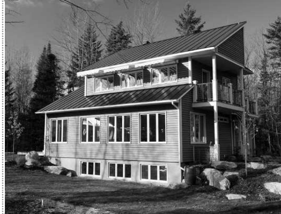
South View of EcoTerra House
