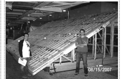
BIPV/T Roof Construction
