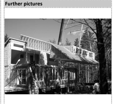
Assembling the prefabricated modules
