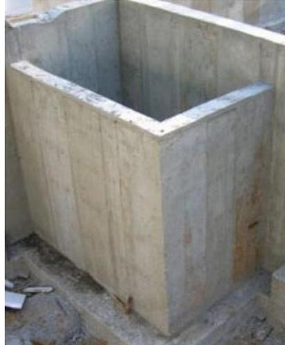
**Figure 4.17.** TES Tank (before insulation was applied).
