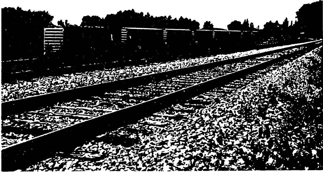
Figure 1.1 Railway vehicles and tracks
