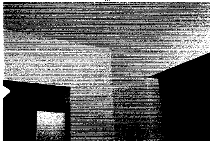
Figure 2.14 Thermogram showing the distribution of surface temperature (a) due to surface coefficient and (b) thermal bridges at the junction of partition walls and roof
