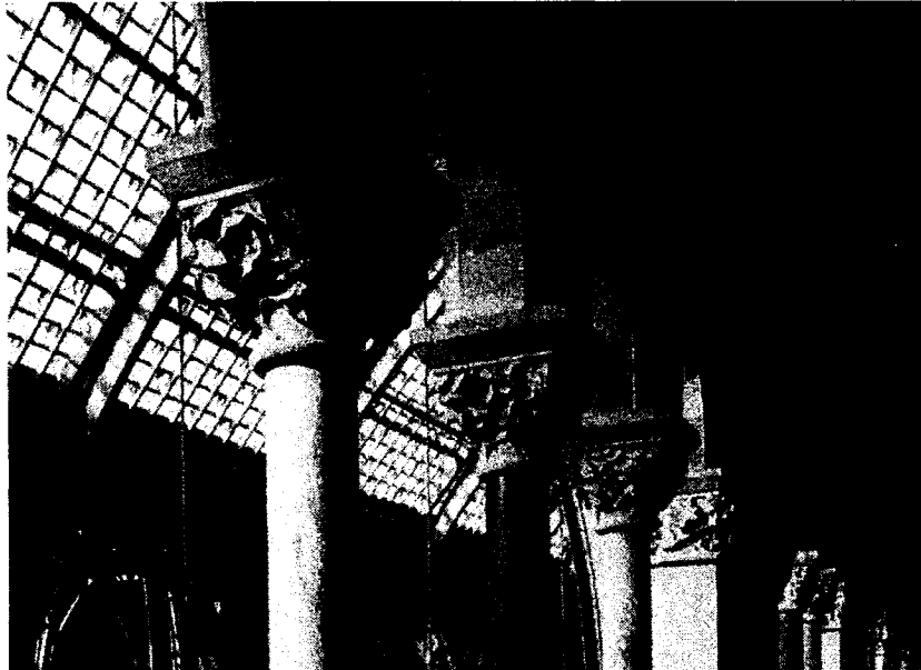
Upper gallery colonnade, Oxford University Museum. Note the different materials for each of the columns and the different design of each of the capitals, which were carved to represent the flora and fauna of Britain.
