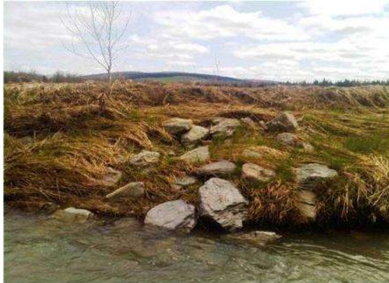
Figure 5.11 Rip Rap as bank fortification on the left bank in zone 2.
