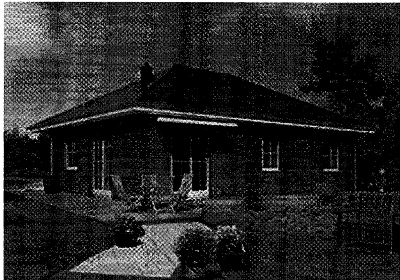
Figure 3.6: Typical bungalow residential building with brick cladding (CREA, 2006)
