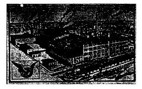
4-18t: Island City Paint and Varnish Works; Note the prominence accorded to the factory's ability to interact directly with the railway and the water, through large doors at street level.
