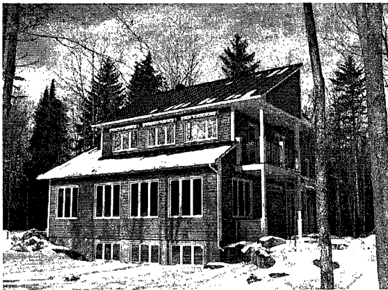
(c) 12:00pm south roof
