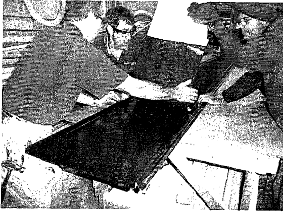
(a) Glue PV panel on metal roofing
