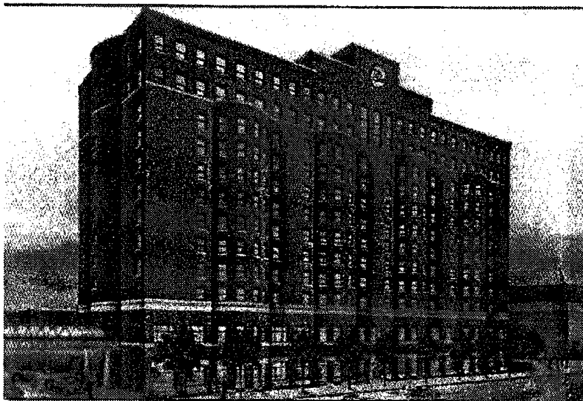
Figure 1.2. Renaissance Hotel, 12-story reinforced masonry building, Springfield, Illinois (Taly (2001))
