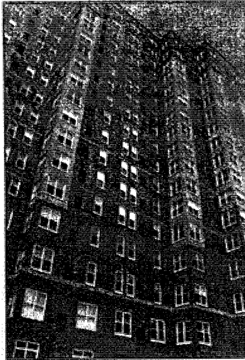
Figure 1.1. The Crittenden Court, 17-story reinforced masonry high-rise, Cleveland, Ohio (Taly (2001))
