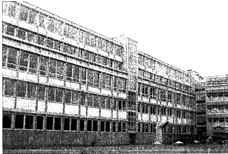
Figure 2.7: The Schwerzenbacherhof Building
