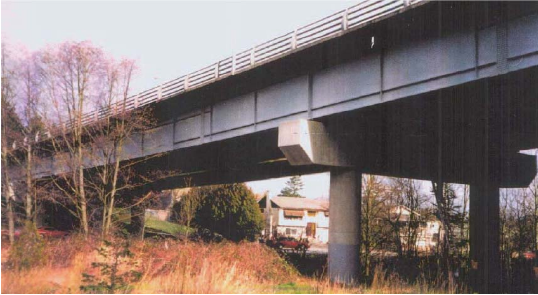
Figure 1: Portage Creek Bridge, Victoria, British Columbia, Canada
