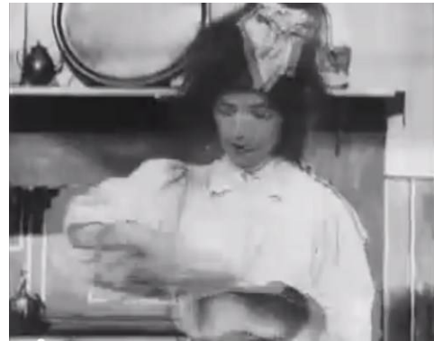
(11.4) Closer framing, revealing more details.
