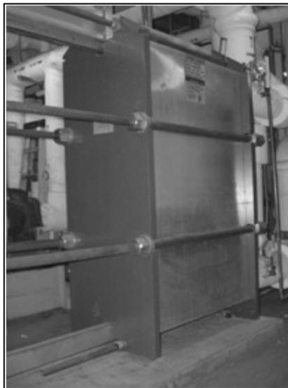
Figure 2-1 Plate heat exchanger
