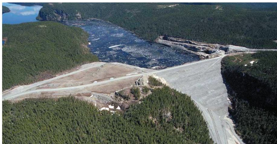
Figure 5.2 The Saint-Marguerite-3 after Construction
