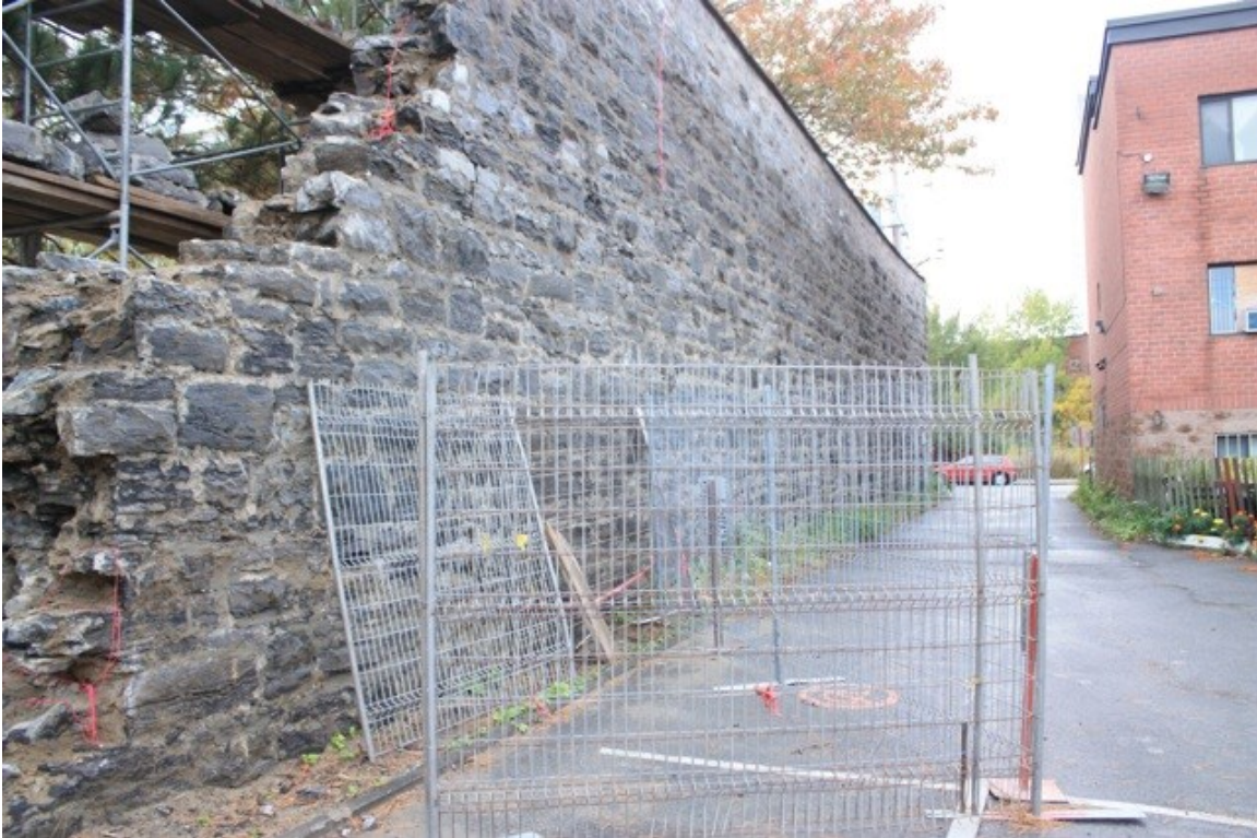
Fig. 8 The Wall of the Convent, 2012
