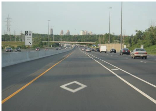
Figure 4: Buffer-separated Concurrent HOV lane (Haljackey (2010))
