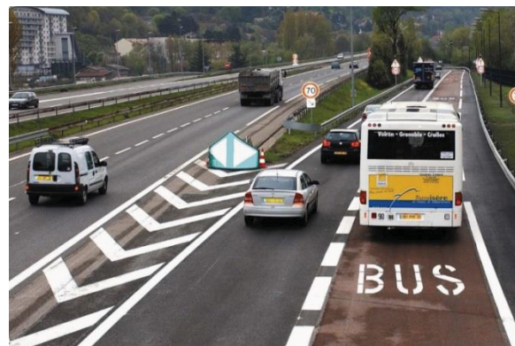
Figure 9: Bus-lane on the right-side of the exit of a freeway near Grenoble (France) (Pollet, et al. (2005))
