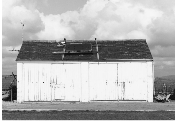
Figure 3.10: Single Storey building used (Sharples & Charlesworth, 1998)
