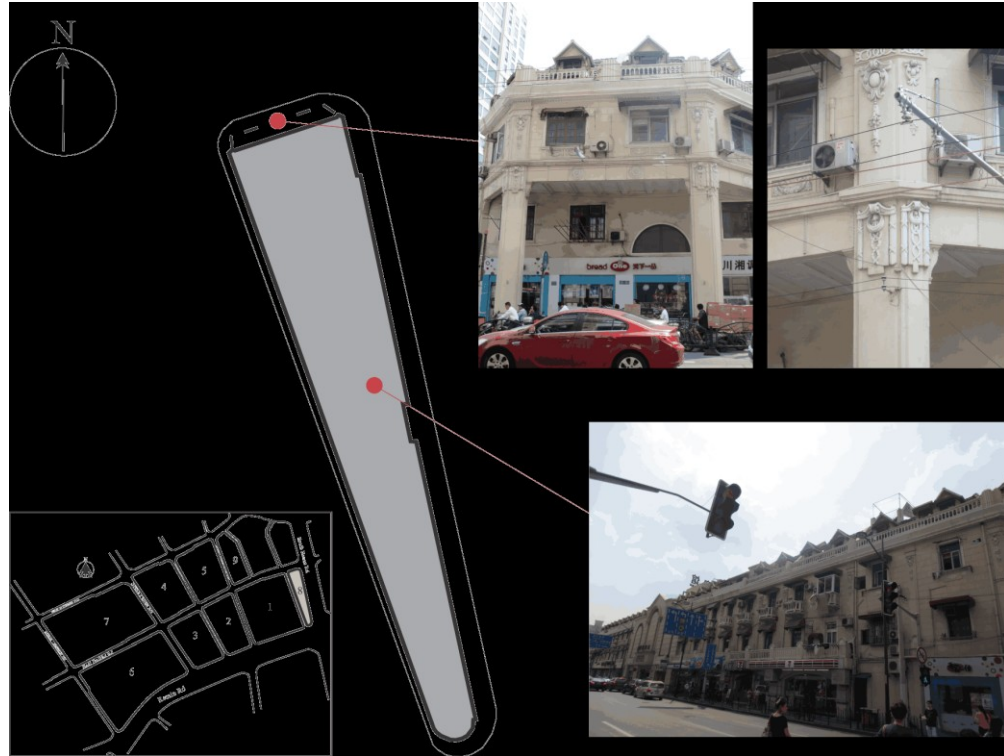
Figure 4-32: Block 8: Shanghai Manhattan Jinling Business Hotel.
